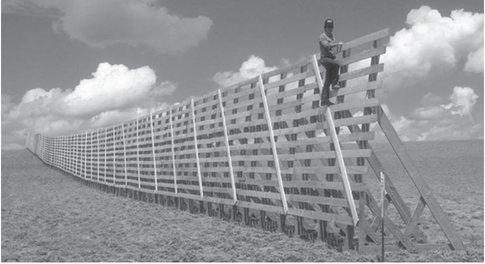
Figure 12.2 Wyoming snow fence that has been extensively tested and used to control blowing snow in Western United States (Tabler 2003, © 2003 by Ronald D. Tabler, all rights reserved. Reprinted with permission).
